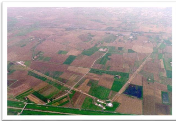
Aerial view of the site construction near Cascina (Italy)
